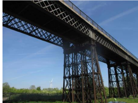
General view of trestles and primary lattice beams
