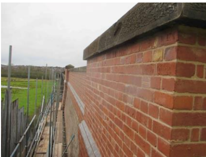
Reconstructed east abutment
