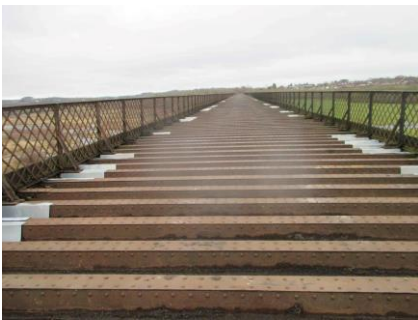
Removed ballast and zinc plate inserts to deck trough ends
