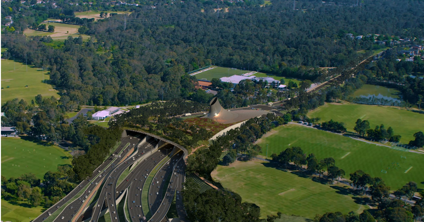
NEL – Contract Close visuals of the Southern Portal: Ventilation Stack and Land Bridge
