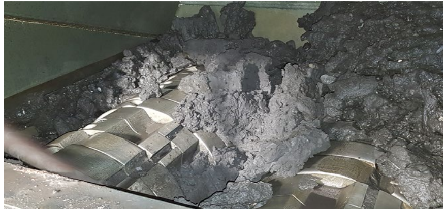
Clogging at sizer box (rotary crusher)
